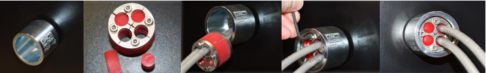
A typical MSR 40 Type 3 being installed
